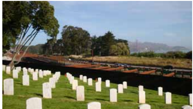
Work on Doyle Drive (2011)
