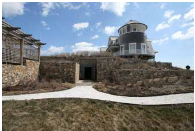
The entrance to Battery 210 at Mishaum Point (Chris Zeeman)
