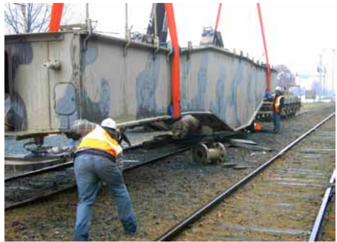
K5 gondola being lifted at APG
