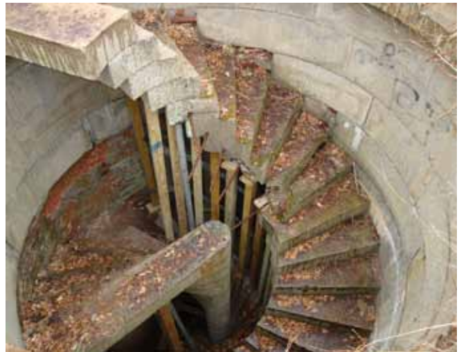
The repaired stairs at the Advance Redoubt (Mark Berhow)
