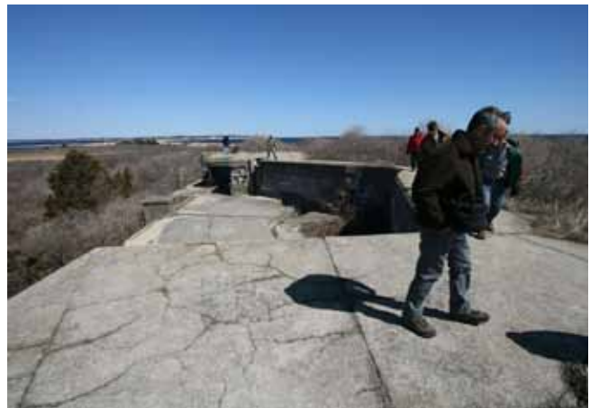
Battery Wooster, Fort Mansfield (Chris Zeeman)
