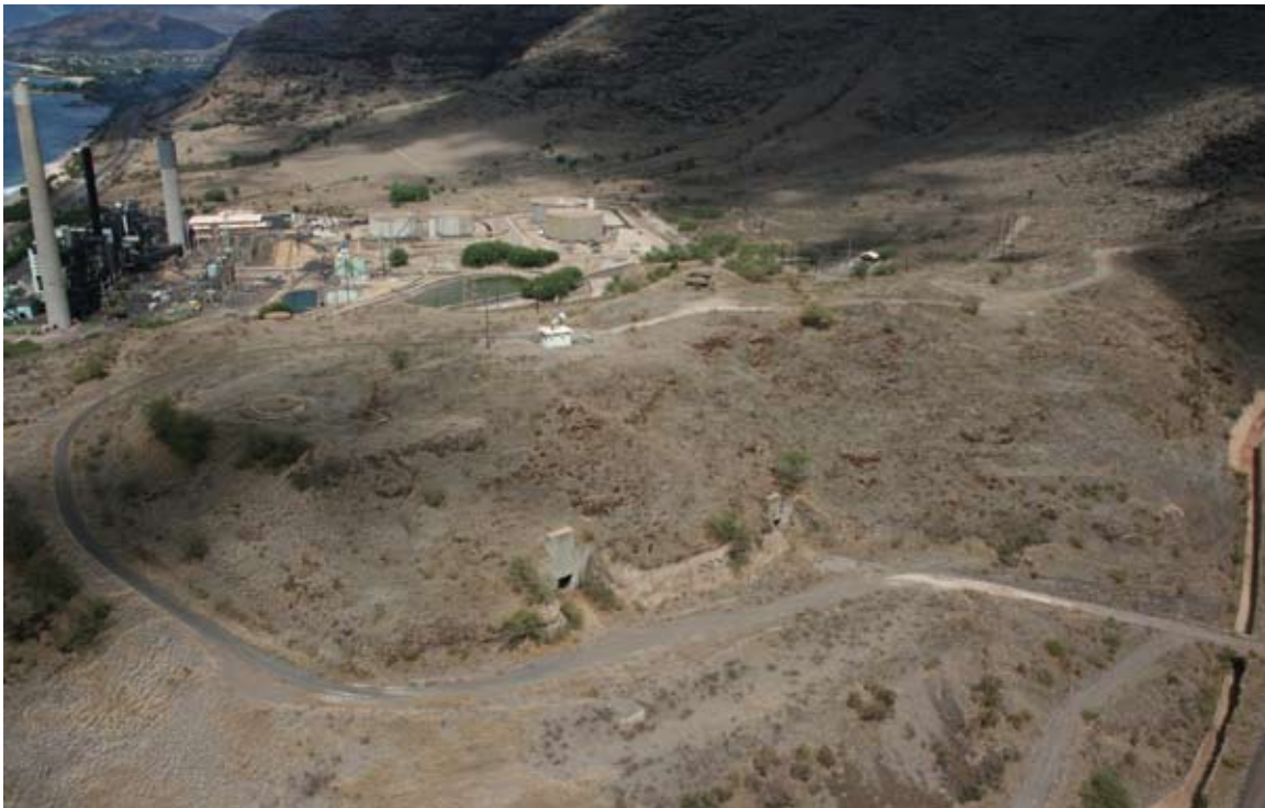
Battery Arizona – Kahe Point (T. McGovern 2009)
