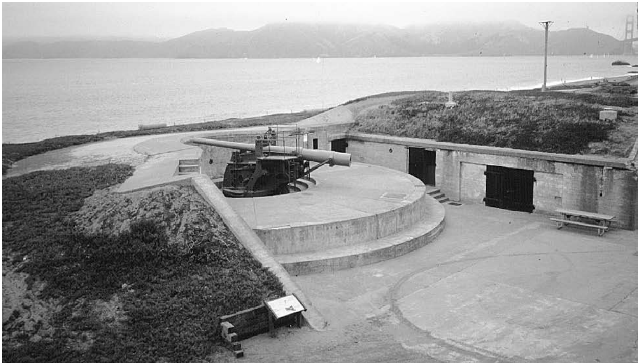
Battery Chamberlin, Fort Winfield Scott, Golden Gate National Recreation Area, San Francisco, California (1994) This battery features a 6-inch gun on a disappearing carriage
